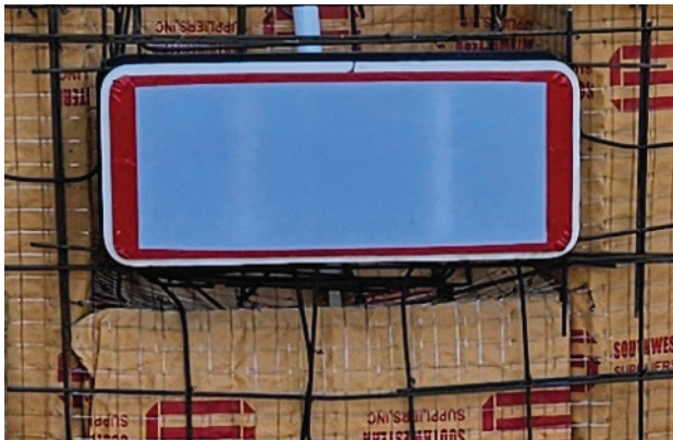
Image 3 Placement in rebar
