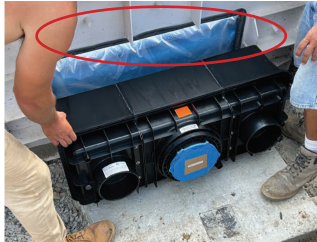
Image 8 Installed butterfly gasket
