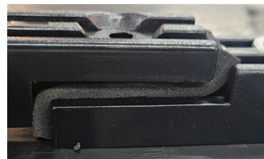
Image 13 Foam Strip Installation
