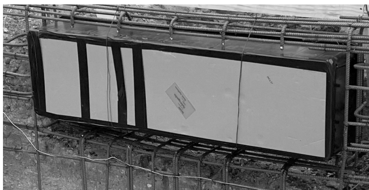
Image 4 BaduJet Turbo - Jet placement in rebar
